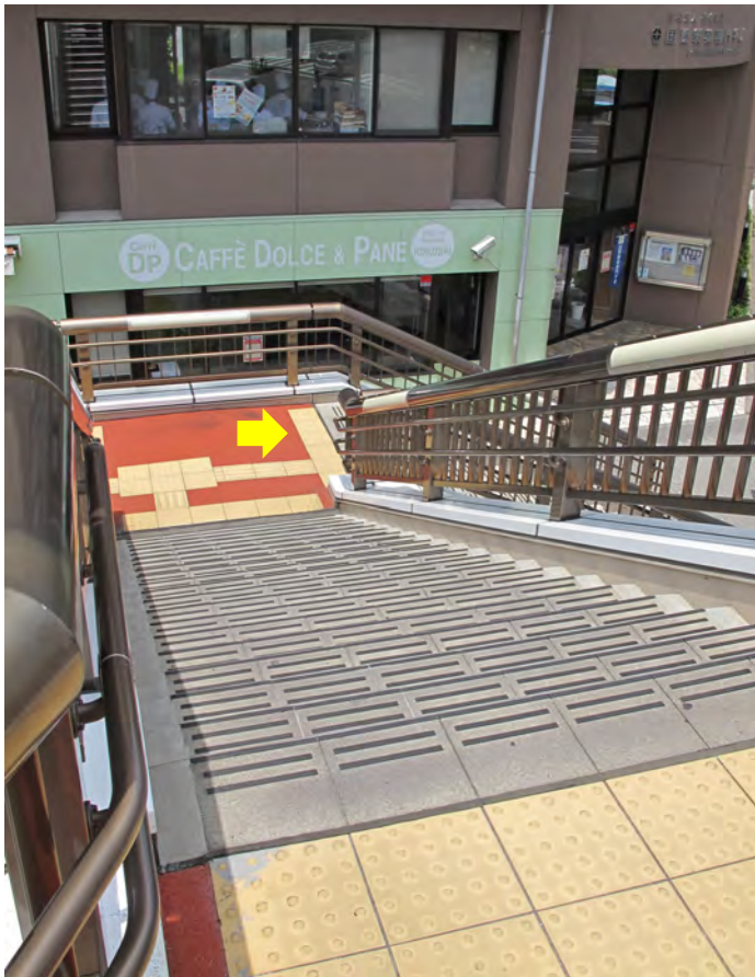
stairway to street level
