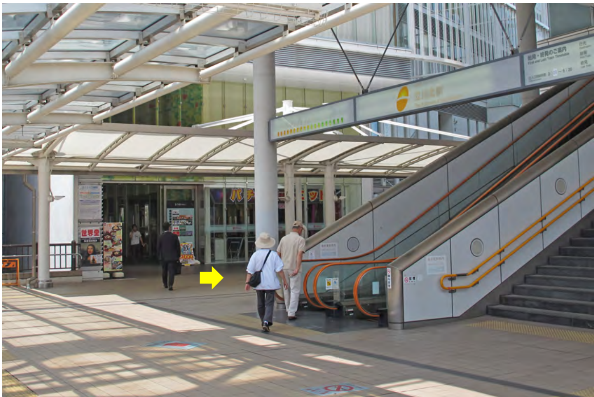
monorail station escalator
