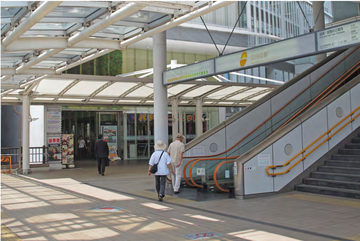
monorail station escalator
