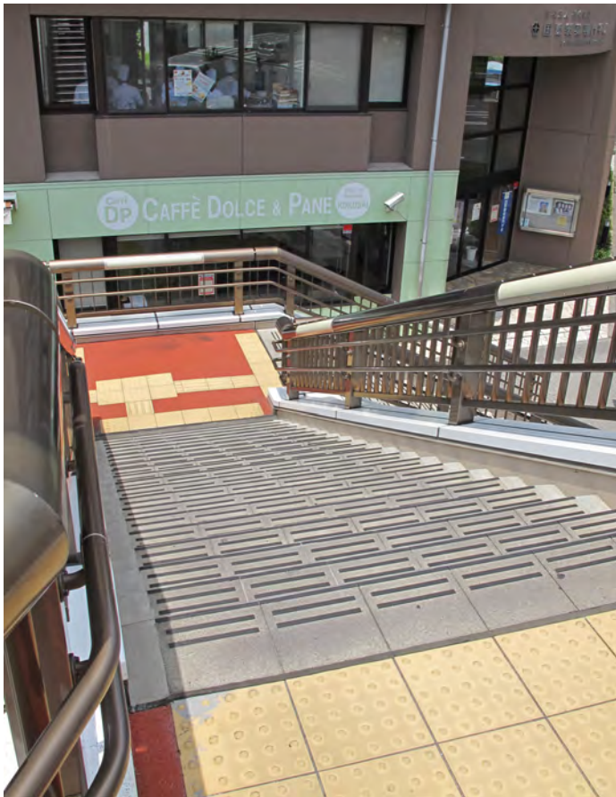
stairway to street level
